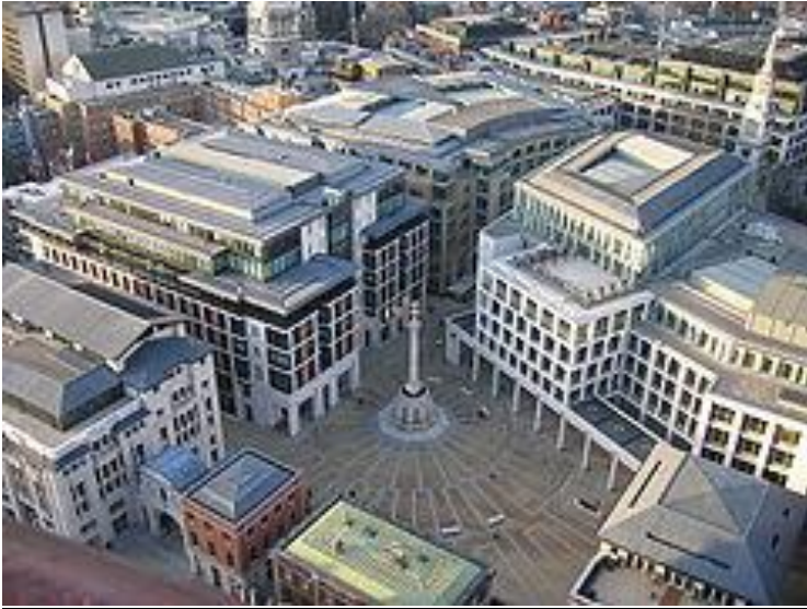
The Stock Exchange building seen on the right
